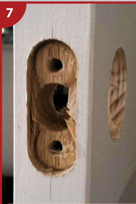
7. Example of 'door preparation' completed - ready for the latch/bolt to be installed.
