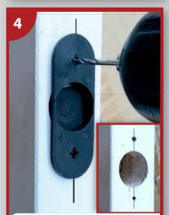
4. Insert the plastic Strikebox/drilling template into the edgebore hole and use as a guide to drill  $2x \not 0$  3mm pilot holes above and below edgebore hole. Insert strikebox/drilling template into the  $\emptyset$  24-25mm hole created in jamb (3a) and drill  $2x \not 0$  3mm pilot holes above and below  $\emptyset$  24-25mm hole.
