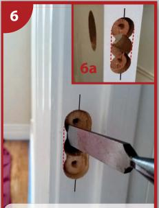
6. Use a blade or pencil to mark vertical lines down the sides of the 3x overlapping Ø 24-25mm holes on door and jamb (6a). Use a Chisel to remove timber from the sides of the overlapping Ø 24-25mm holes where marked.
