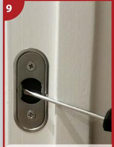
9. Insert the strikeplate assembly (incl. strikebox/drilling te late into the prepared jamb 'cutout' so that the latch/bolt rests against Adjustment Tab A when in the locked/latched position (FIG. C). Secure in place with screws provided. Test door operation and if necessary 'bend out' adjustment tab with the AM60 ITP screwdriver (FIG.B), to reduce latch/bolt rattle
