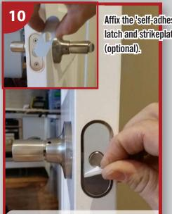
10. Affix the coverplate (A) to the face of the latch/bolt, as shown. Press firmly over the entire surface of the coverplate to ensure maximum adhesion. Remove plastic protective film from surface. Note: make sure metal faces of latch and strikeplate are free from dust /oil etc before affixing coverplates, to insure maximum adhesion strength.
