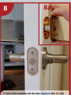
secure in place with screws provided. Be careful not to over tighten screws as this may cause the flanged housing cups to deform and/or cracking in timber. Note: screwheads must fit below, or perfectly flush to the surface of the latch/strikeplate, to allow coverplates to adhere properly to surface (FIG. A). Now install chosen door handles as per manufacturers instructions.
