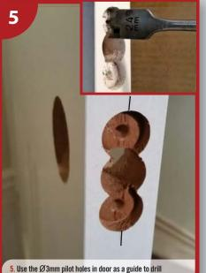
5. Use the Ø3mm pilot holes in door as a guide to drill 2 x Ø24-25mm overlapping holes (above and below the edgebore Ø24-25mm hole) to a depth of approx. 5mm. Repeat this step on the jamb to create 2 x overlapping Ø 24-25mm holes.
