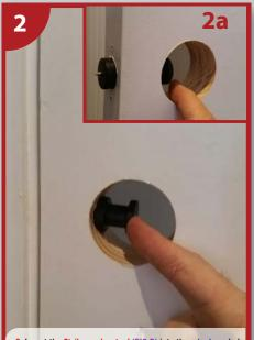
2. Insert the Strikemarker tool (FIG.B) into the edgebore hole (2A). Close door tightly then press the pointed Strikemarker tool
