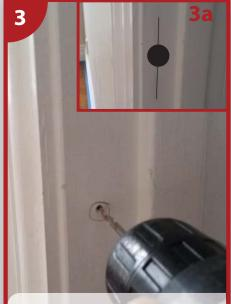
3. Drill a Ø 3mm pilot hole into the jamb at the position marked by the pointed Strikemarker tool. Use the pilot hole as a guide to drill a Ø 24-25mm hole into the jamb to a depth of approx. 20mm (3a).
