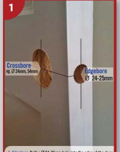
1. Edgebore-Drill a Ø 24-25mm hole into the edge of the door at the desired height. Crossbore-Drill hole(s) into the face of the door at a backset of 60mm to the diameter(s) etc. specified on the chosen
