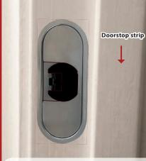
Affix the 'open sided' coverplate (B) to the face of the strikeplate with the open side facing away from the doorstop strip as shown. When correctly fitted, the latch/bolt should not make contact with the coverplate as it engages into the strikeplate.
