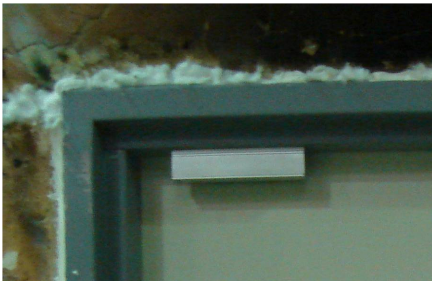
FSH MEM2400M Magnetic Lock Fitted to Doorset in BWA 2209801 Size 158mm x 30mm x 30mm
